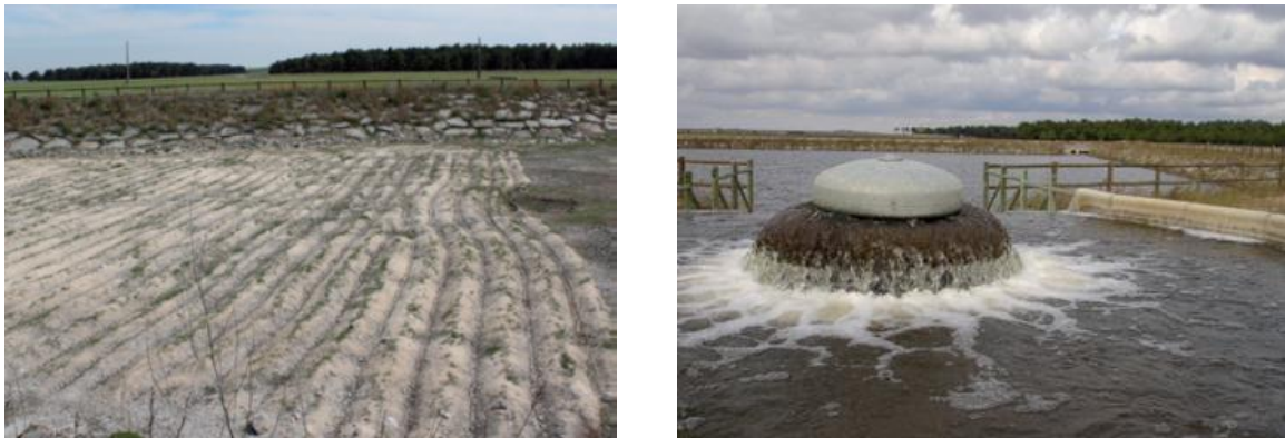
Figure 5 Pictures of infiltration pond bottom surface and flooding process in Santiuste (Spain).
